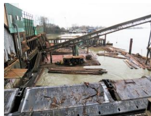
Pulling logs from the river
